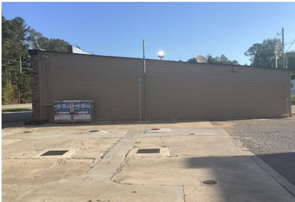
Existing Convenience Store w/Fuel (South Elevation)
