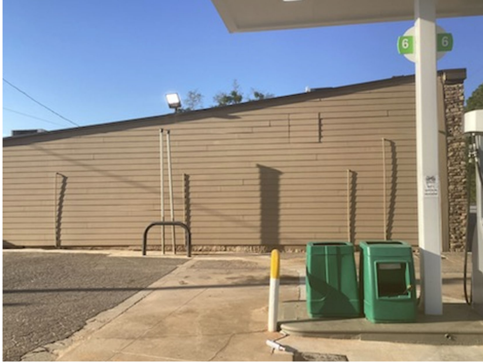
Existing Convenience Store w/Fuel (North Elevation)
